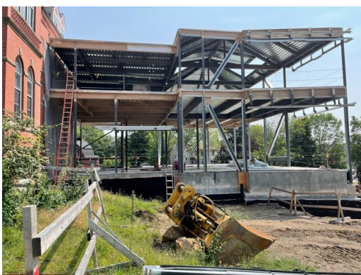
1. Overall Structure, view of fireproofing in progress.
