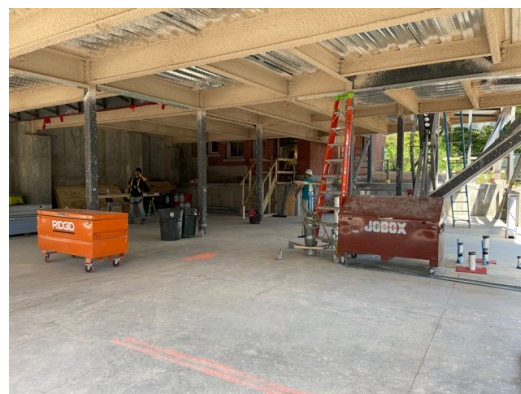
2. View of Lower Level fireproofing.
