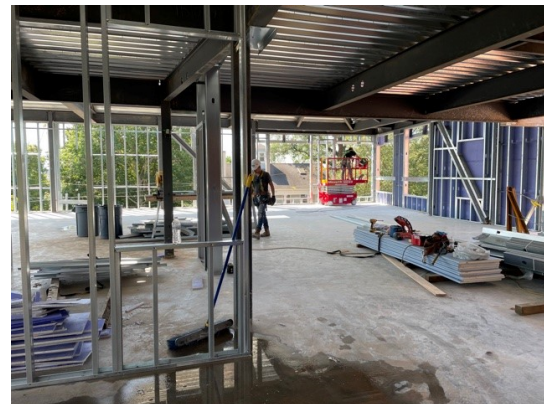
8. View of interior framing beginning in new addition.
