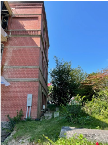
5. View of demolished fire escape.
