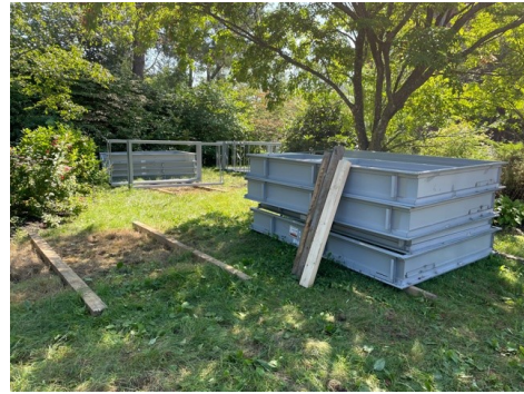
4. Door frames on site.
