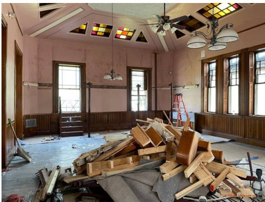
7. Second floor mezzanine demolition.
