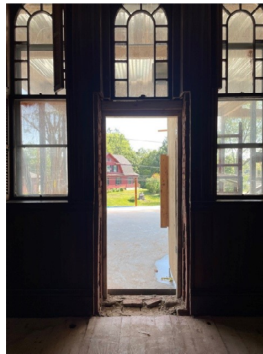
6. View of demolished window for new door opening.
