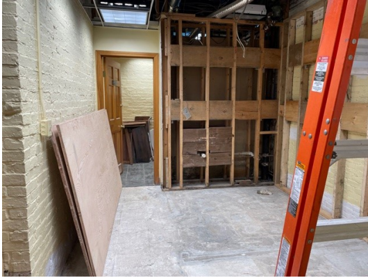
3. Select demo in existing building continues.
