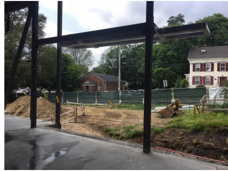
4. View of new entrance from interior.
