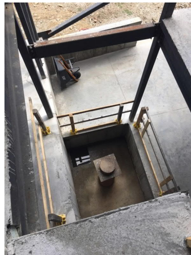
6. View down new elevator shaft.
