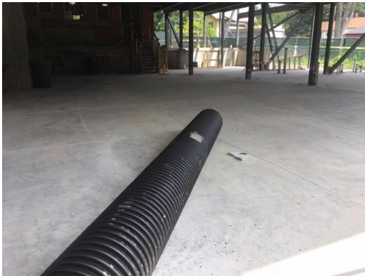
5. View of Lower Level slab.
