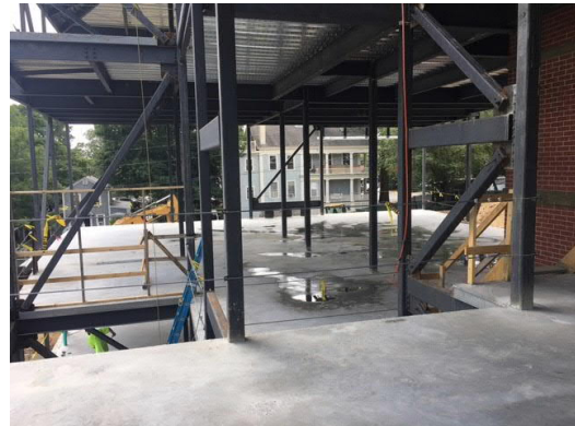
2. View of First Floor concrete slabs.
