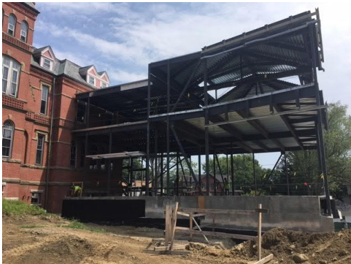
1. Overall Structure, decking and concrete slabs complete.
