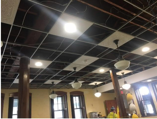
3. Select demo in existing building underway.
