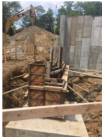
2. Northwest corner of addition: Footing and wall below Community Rooms.
