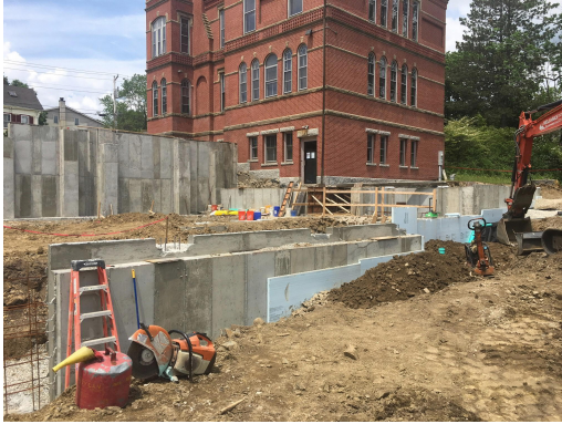
3. South side: foundation and insulation below storage, toilets, and Stair A.
