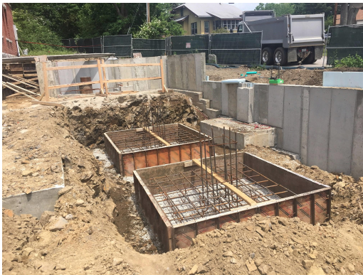
5. South side: Footings for columns at the toilets.
