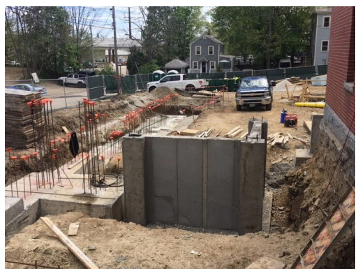
8. East side: Elevator shaft.
