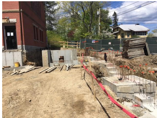
6. South side: Footing below toilets and stair.
