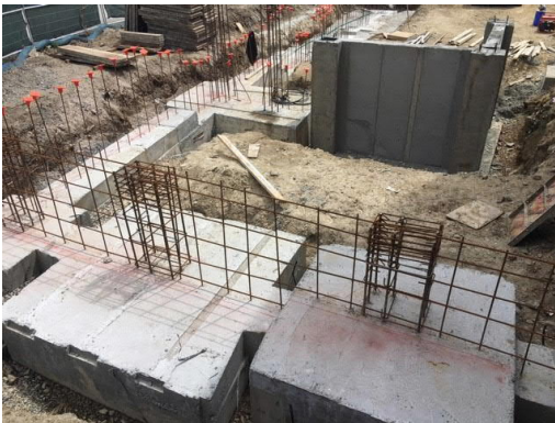
7. East side: footing below Maine Room and Collection.
