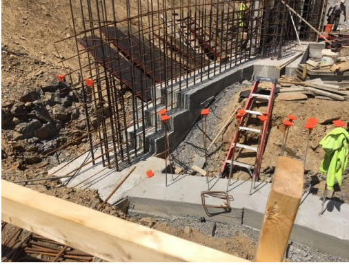
3. Northwest corner: footing below Community Room.
