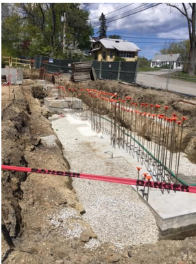
5. South side: Footing below meeting room and toilets.
