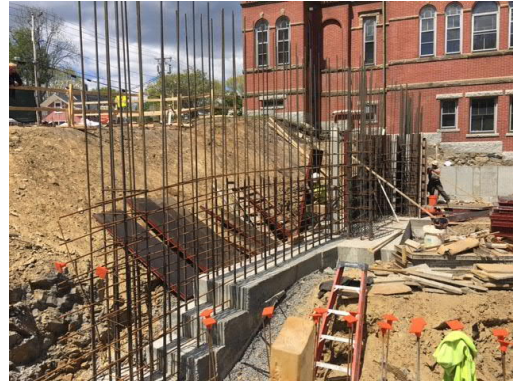
4. North side: footing below Community Rooms.
