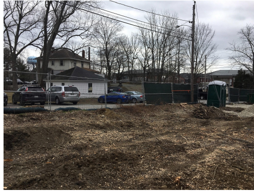
4. Exterior: southeast corner of site looking south.
