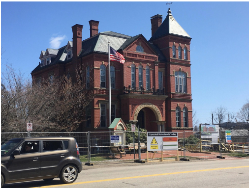
5. Exterior: Signage is up out front indicating daily noise levels.
