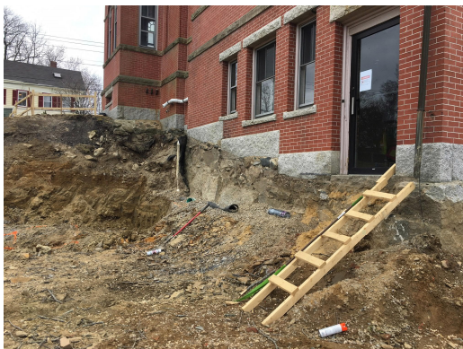
1. Exterior: south corner of site looking north.
