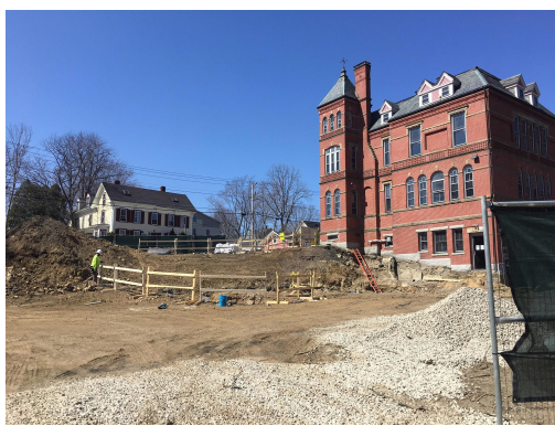
8. Excavation is barricaded off with fall protection.
