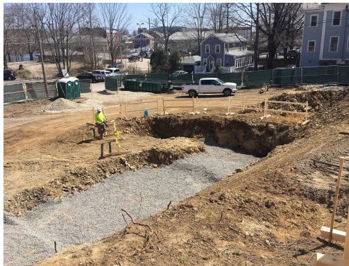
6. Excavation is underway for the addition's foundation.
