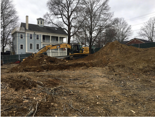
3. Exterior: southeast corner looking northwest.
