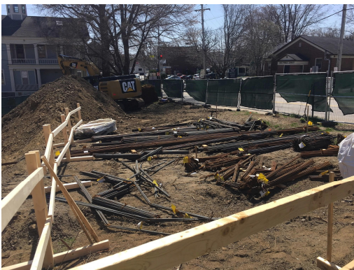
7. Exterior: Rebar for the foundation has arrived on site.
