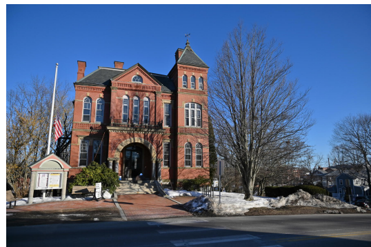
2. Exterior: front façade
