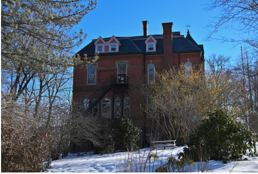
3. Exterior: west façade.
