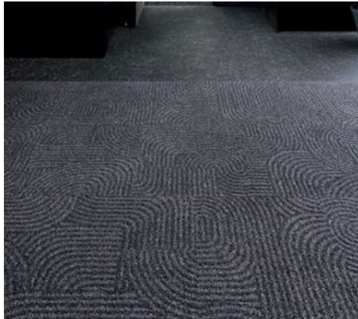
LVT To Carpet Community Room
