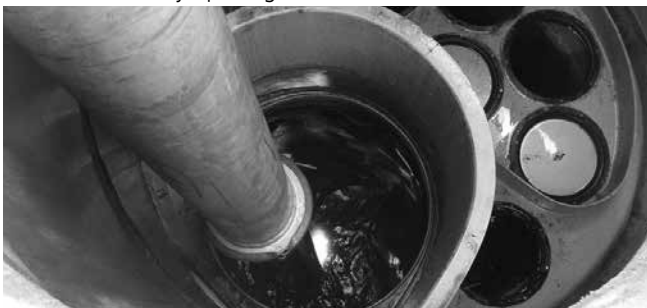
Vacuuming Sump Through MAW
