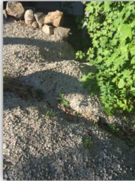
Figure 2. Stormwater from the southeast corner of the house is rapidly released from the gutter, causing erosion.
