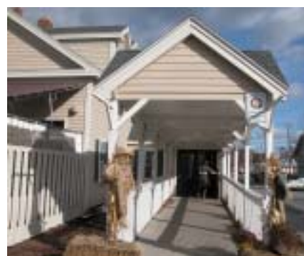
The 9:12 pitch on the shelter covering this access ramp matches the slope on the main roof on this restaurant.
