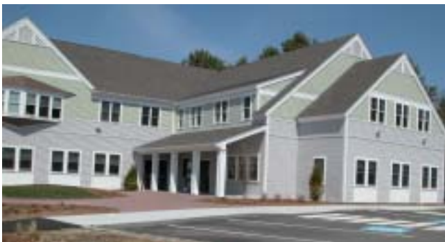
An office building featuring a variety of gable roofs. The pitch on the flat dormer matches the pitch on the entryway.
