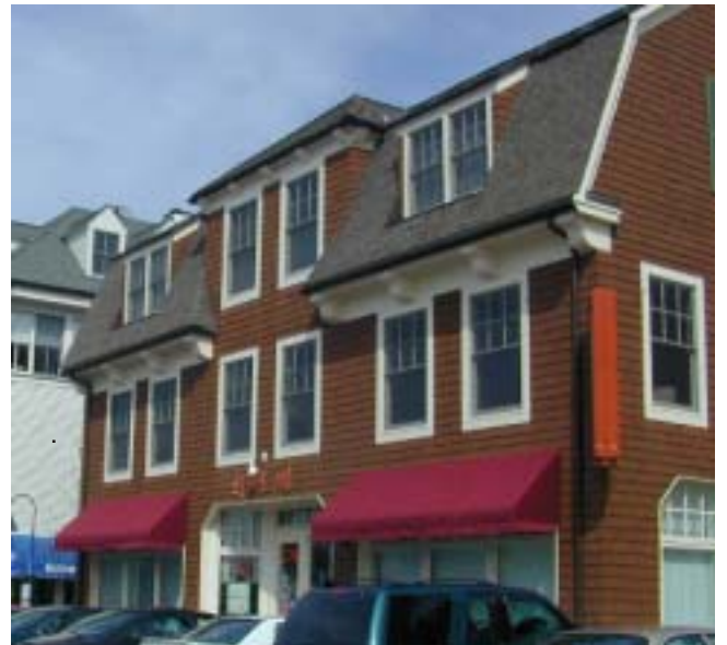
Stained/painted wooden clapboards and cloth awnings
