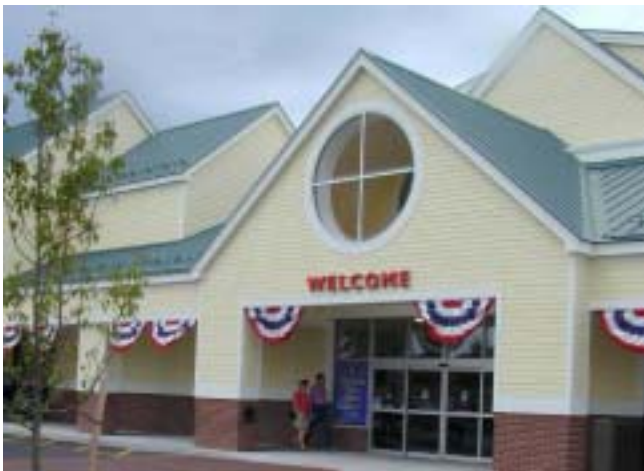
Clapboard siding with brick
