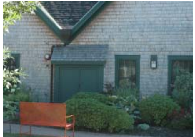
The building's meters and service connections are located out of sight in this service cabinet.
