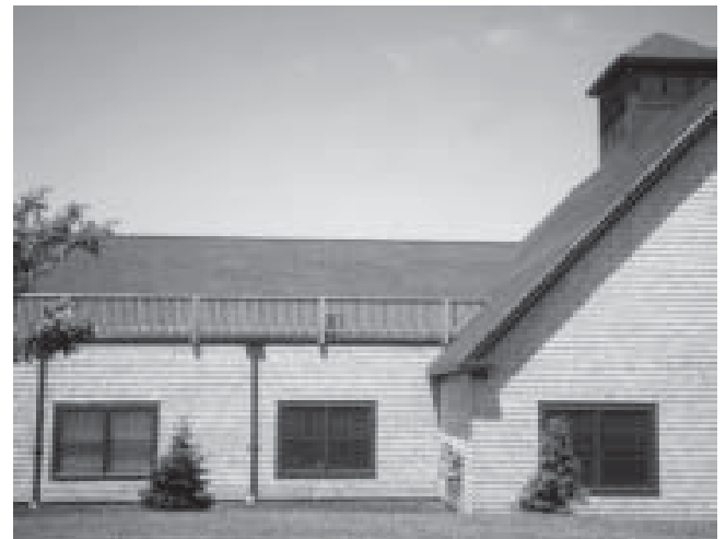
A cupola at the peak of this roof is a traditional form used in a contemporary structure. Roof-mounted mechanical equipment has been effectively screened by balustrades.
