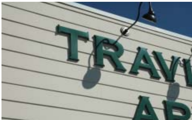
Cement plank clapboard is a new material that resembles traditional wooden siding with less maintenance.
