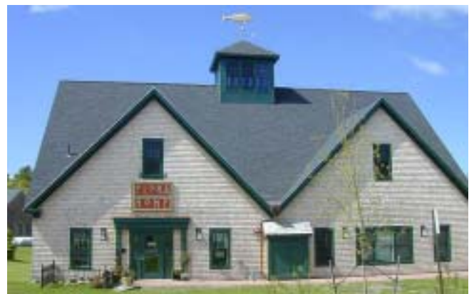
Stained clapboards with wooden cupola
