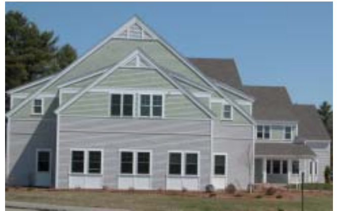
Clapboards with wood panels under windows
