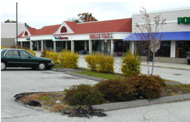
While asphalt curbing is inexpensive to install, it is very vulnerable to snowplow damage.
