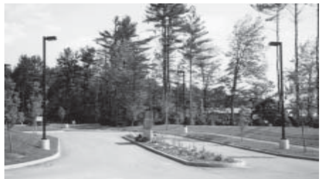
This curbed, landscaped island divides entering and exiting traffic. The identification sign is located away from the intersection to avoid interfering with the motorists' line of sight.
