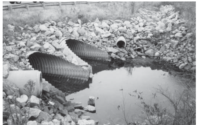
Rip-rap is often necessary to control erosion and stabilize slopes. Hand placed stone or natural landscaping would have improved the appearance of this treatment pond.
