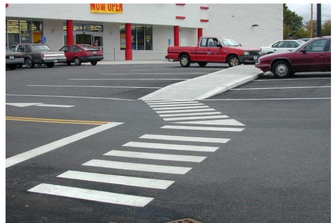
This raised walkway provides a high level of contrast with the surrounding parking lot. However, the width is compromised by the overhang of cars, making pedestrian movement difficult.
