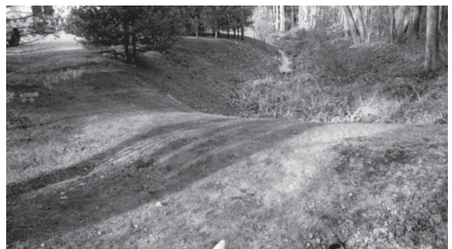
A stormwater treatment facility that is contoured to blend into the surrounding landscape.
