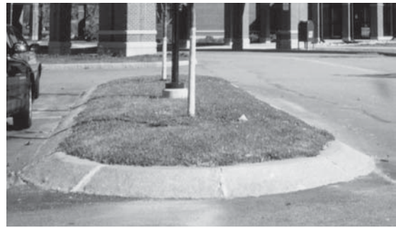
Parking lot islands should be defined by durable curbing materials to protect trees and minimize maintenance.
