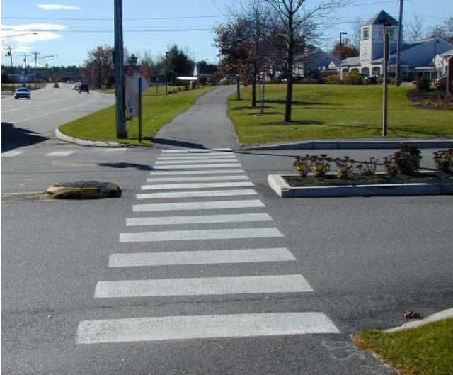
An island provides a refuge zone for pedestrians crossing this wide driveway. Permanent crosswalks should have minimized annual maintenance costs.
