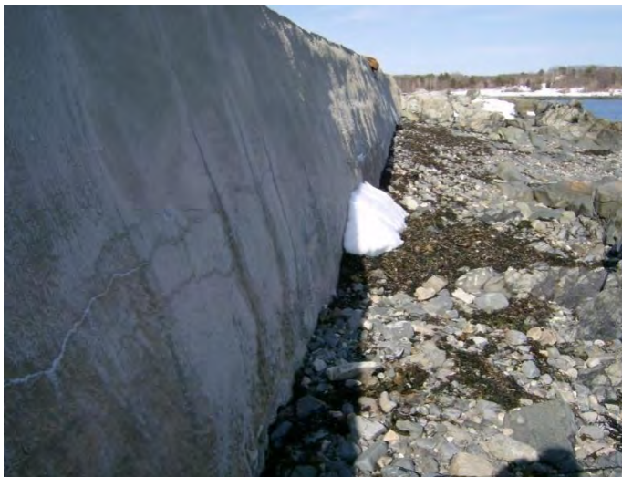
Figure 30: High Tide Marks on South Seawall (2)
