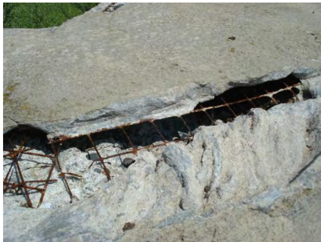
Figure 19 Damaged top section of south seawall
