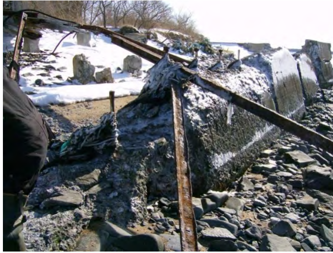
Figure 45: Corrosion of Tie Anchors along North Seawall (2)
