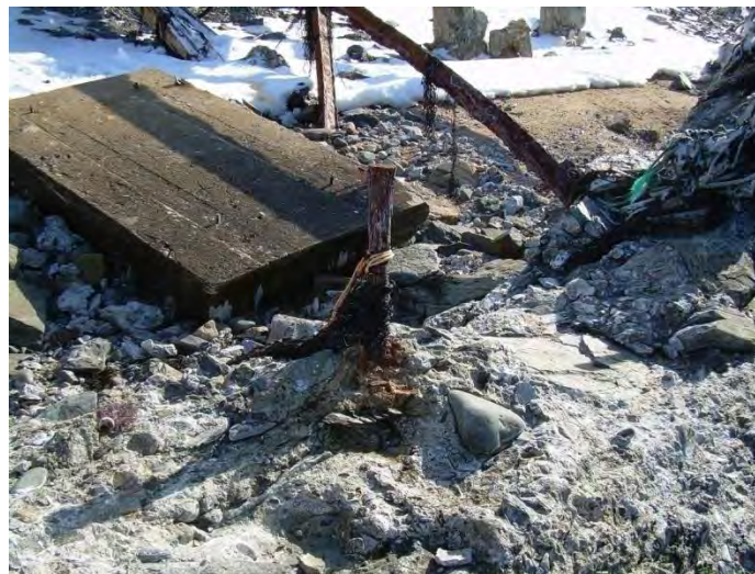
Figure 44: Corrosion of Tie Anchors along North Seawall (1)
