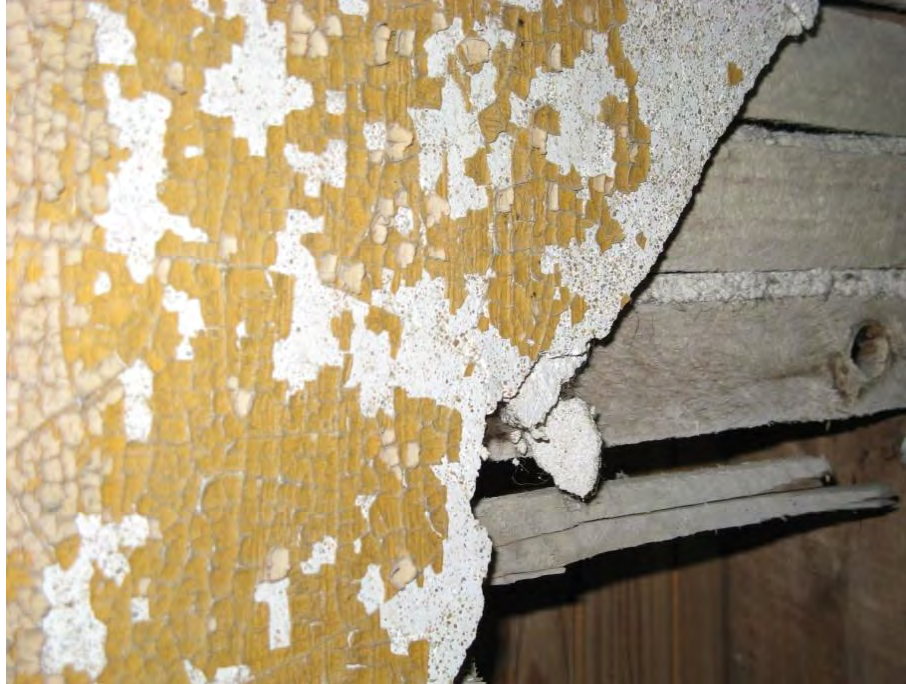
Figure 5: Lead paint chipping off interior walls
