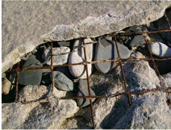
Figure 22: Un-bonded Shotcrete Cap of South Seawall with Gravel Fill
