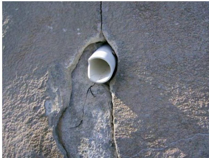
Figure 26: Weephole located halfway up on South Wall
