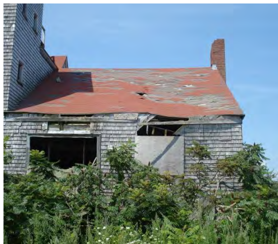
Figure 9: Damage to roof in July 2008
