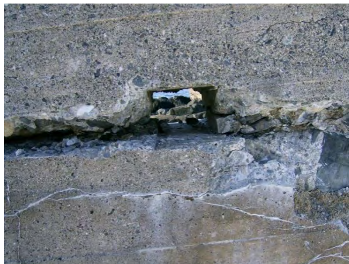
Figure 43: Cast in Place Drainage along North Seawall
