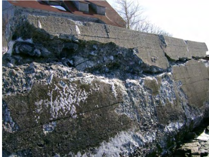
Figure 39: Freeze Thaw Action on North Seawall
