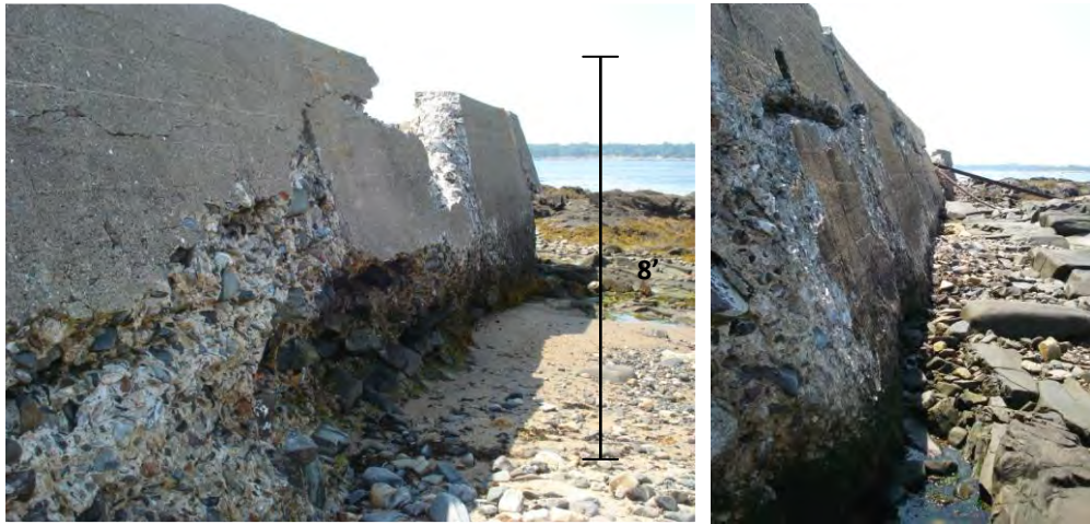
Figure 21 Outer north seawall damage
