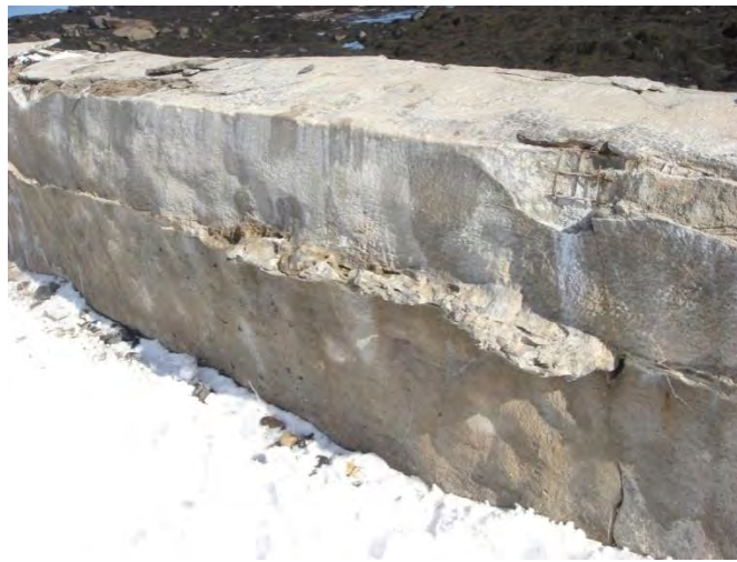
Figure 28: Signs of Backfill Weathering
