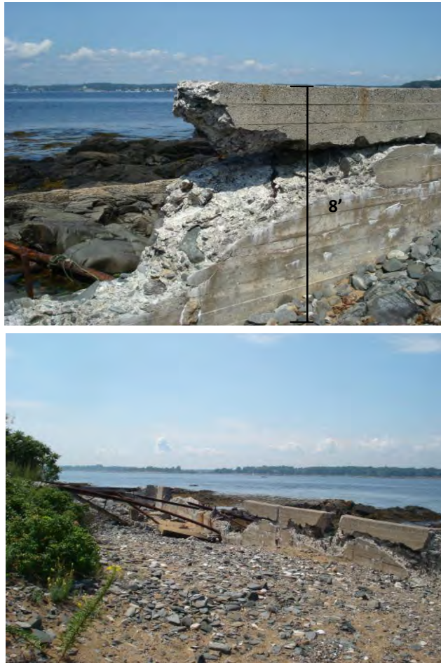
Figure 20 Inner north seawall damage
