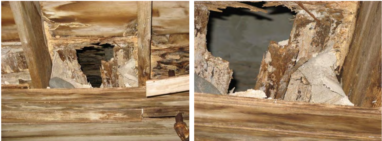
Figure 4: Paper liner within the floors that has been deemed suspect material
