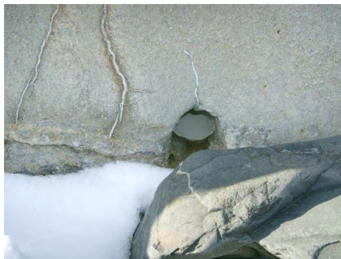
Figure 27: Weephole at toe of South Wall
