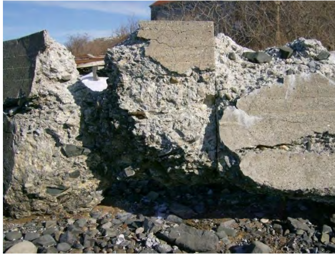
Figure 34: Undercutting of North Seawall (1)
