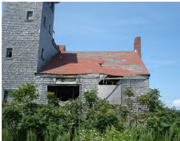
Figure 6 Collapsed station roof
