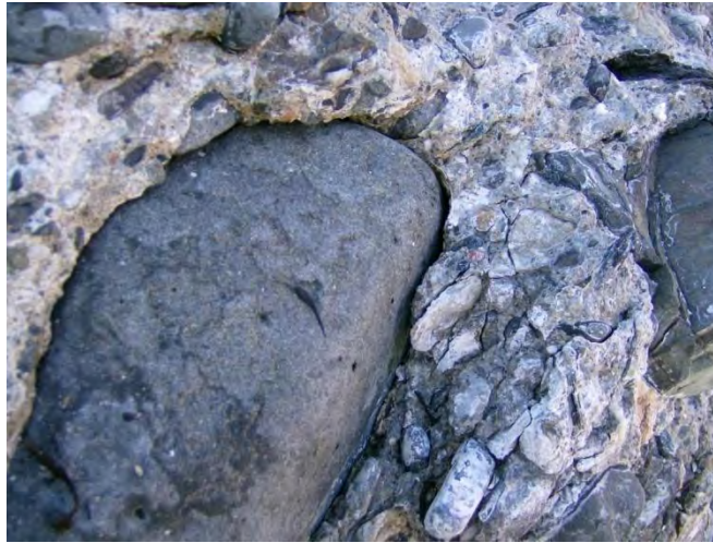
Figure 41: Un-bonding of Aggregate due to Freeze Thaw in North Seawall
