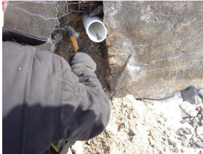
Figure 24: Chiseling into Original Wall near Weephole Weathering
