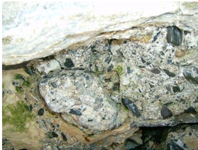
Figure 19: Undercutting of South Seawall
