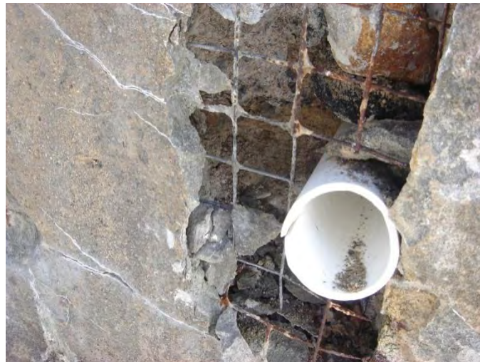
Figure 22: Un-bonded Shotcrete Cap of South Seawall with Gravel Fill
