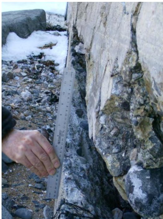
Figure 36: Horizontal Displacement and Overturning of North Seawall (1)
