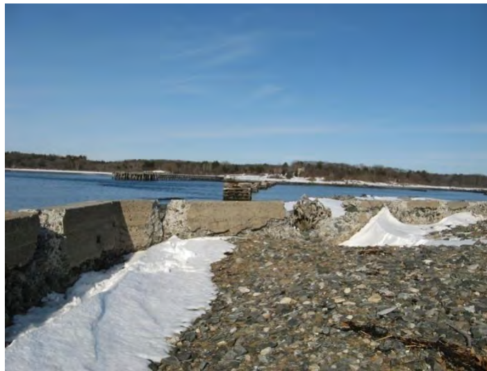
Figure 38: Weathering at Locations of Construction Joints along North Seawall
