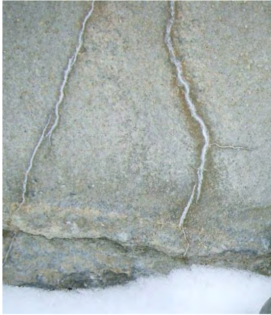
Figure 33: Leaching of Sulfates from South Seawall
