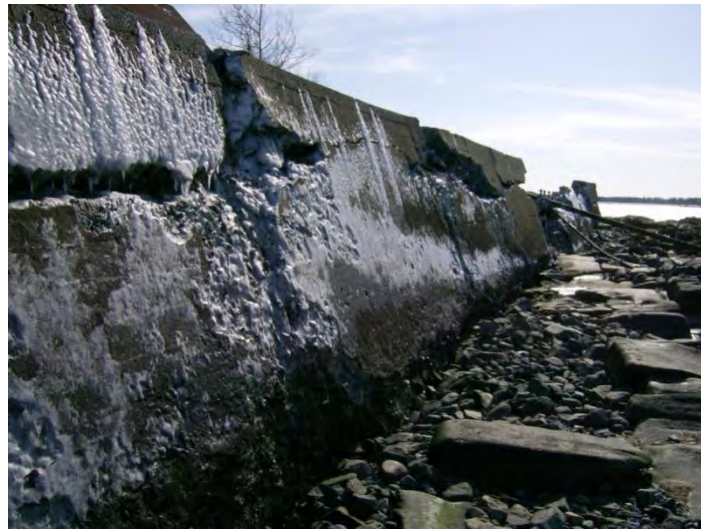
Figure 40: Visible Freeze Thaw on North Seawall
