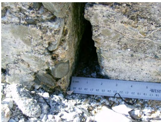
Figure 37: Horizontal Displacement and Overturning of North Seawall (2)
