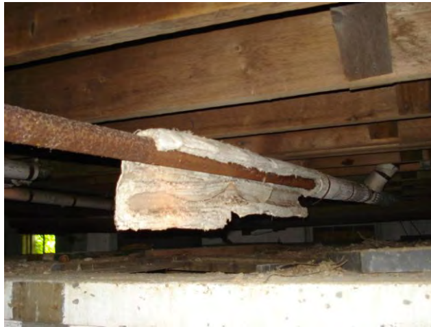
Figure 12 Fibrous pipe insulation
