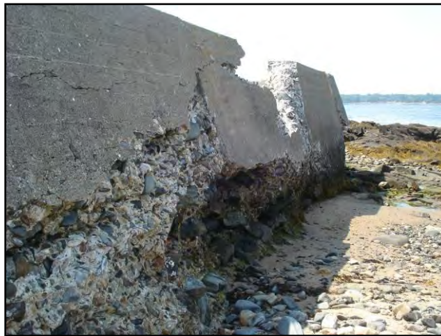
Figure 35: Undercutting of North Seawall (2)
