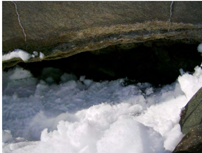
Figure 19: Undercutting of South Seawall
