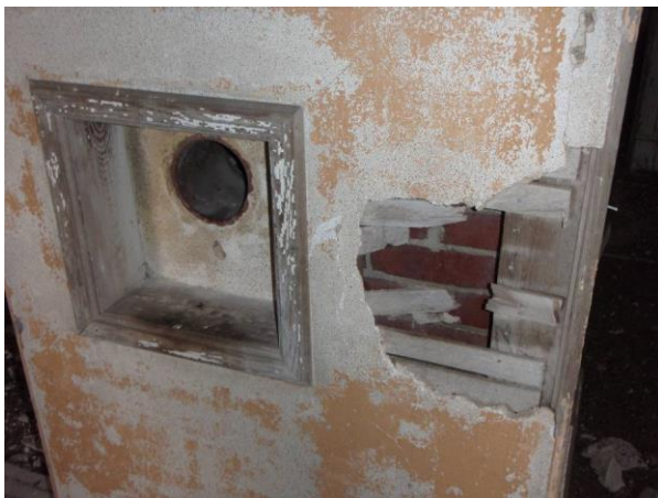
CHIMNEY/THIMBLE – 2ND FLOOR (WEST)
