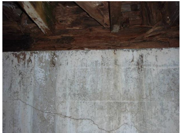
FOUNDATION WALL CRACKS/DAMAGED SILL
