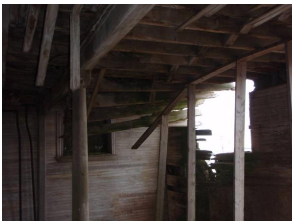
COLLAPSED SOUTHEAST SECTION
