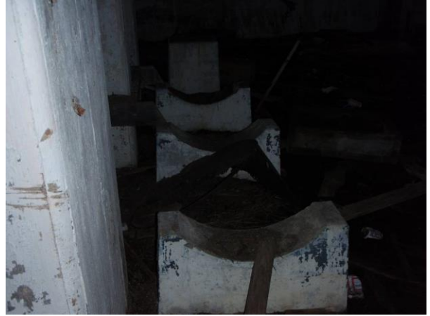
STORAGE TANK CRADLE - BASEMENT
