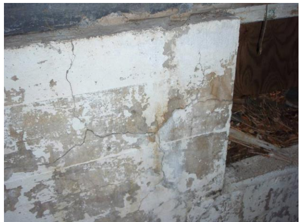
FOUNDATION CRACKS – EXTERIOR
