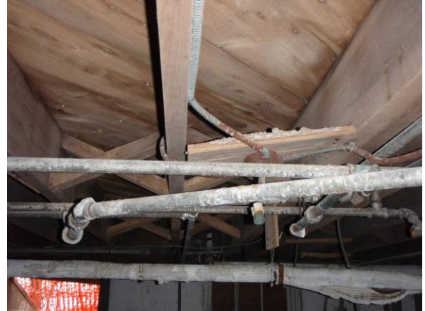
BASEMENT – ASBESTOS LAGGING
