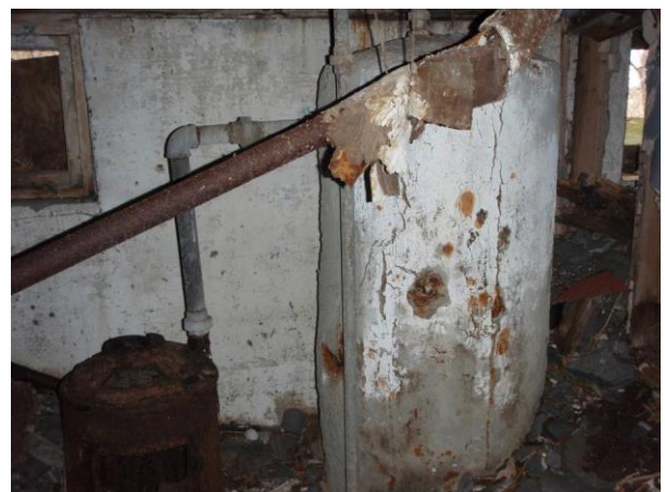
ASBESTOS LAGGED HOT WATER TANK
