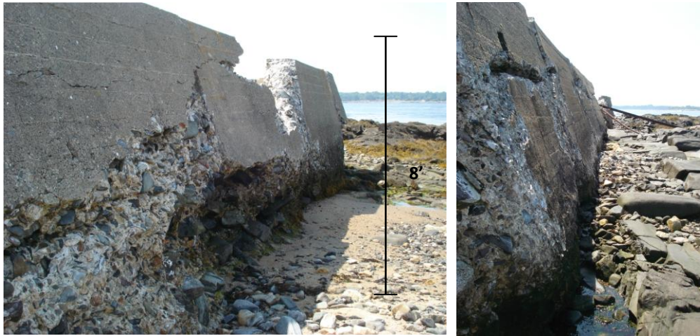
Figure 21 Outer north seawall damage
