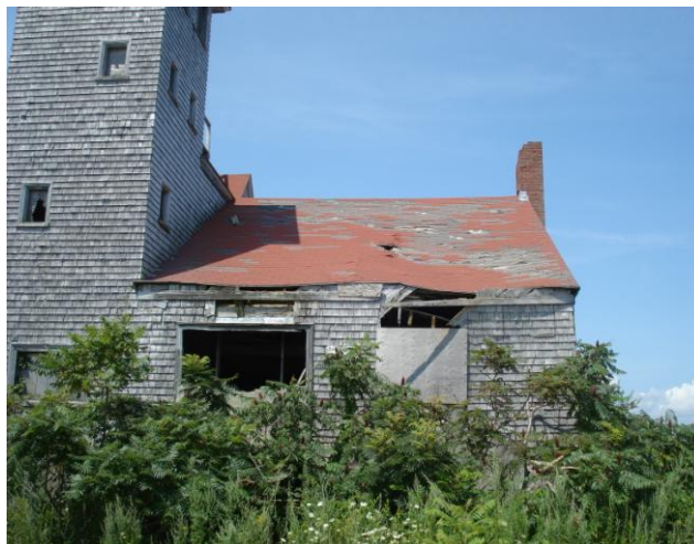
Figure 6 Collapsed station roof
