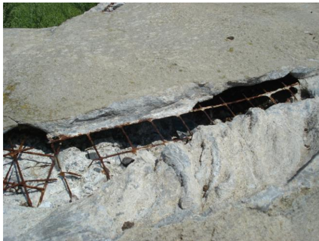
Figure 19 Damaged top section of south seawall
