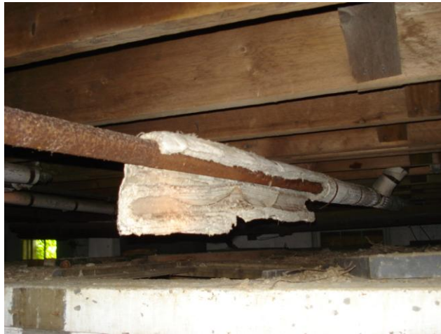
Figure 12 Fibrous pipe insulation
