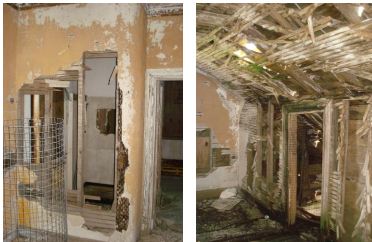
Figure 9 Non-structural interior damage
