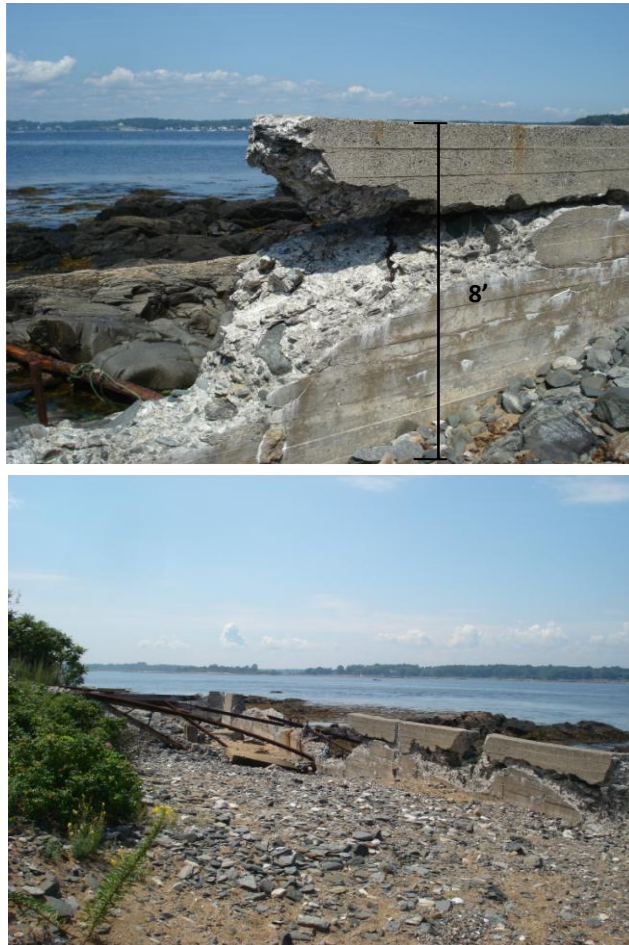
Figure 20 Inner north seawall damage
