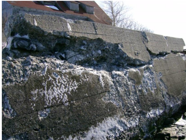
Figure 39: Freeze Thaw Action on North Seawall
