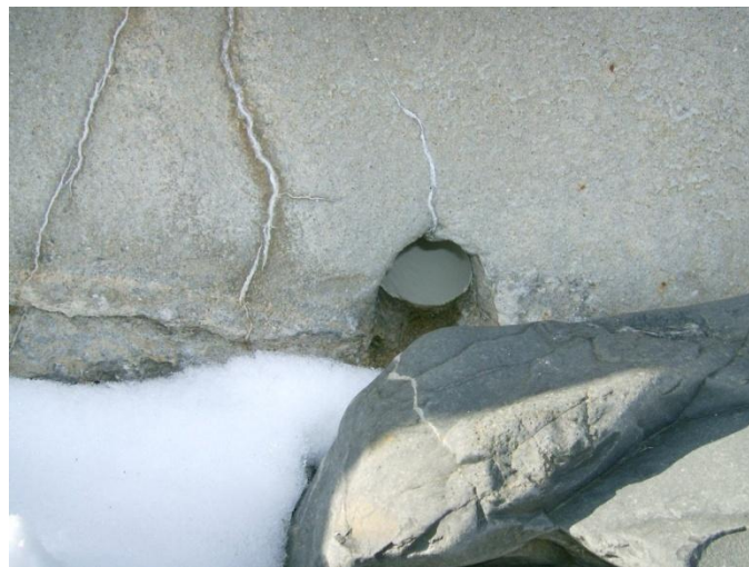
Figure 27: Weephole at toe of South Wall
