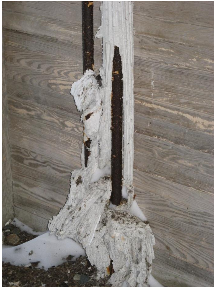
Figure 3: Piping with suspect asbestos containing material used as insulation
