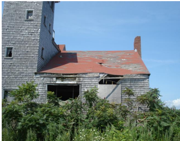
Figure 6 Collapsed station roof
