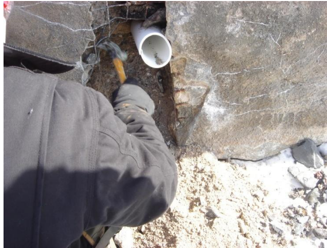
Figure 24: Chiseling into Original Wall near Weephole Weathering
