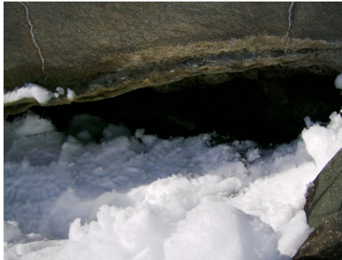
Figure 19: Undercutting of South Seawall
