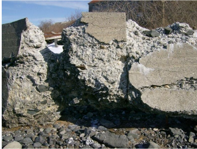
Figure 34: Undercutting of North Seawall (1)
