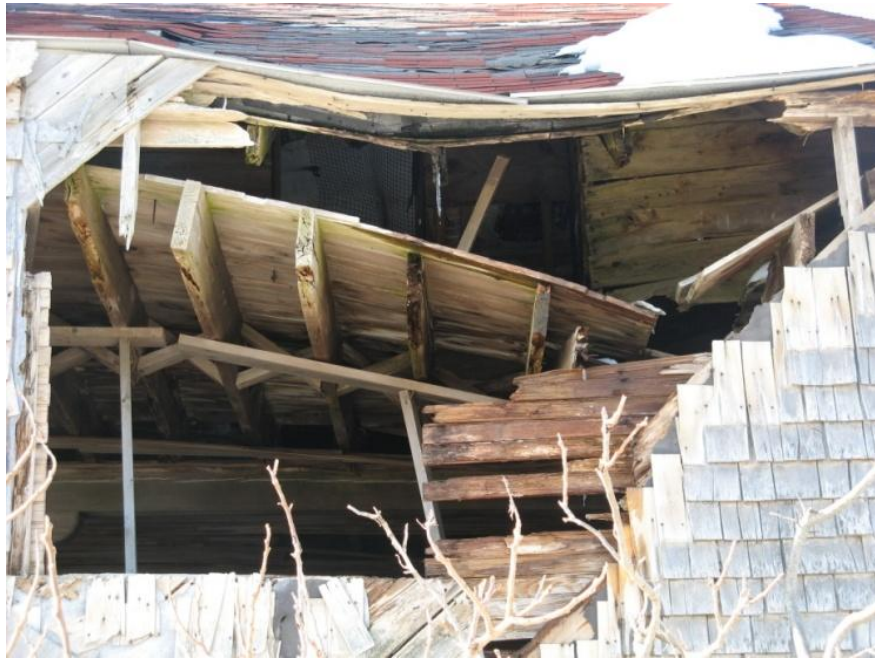
Figure 2: Damage near openings
