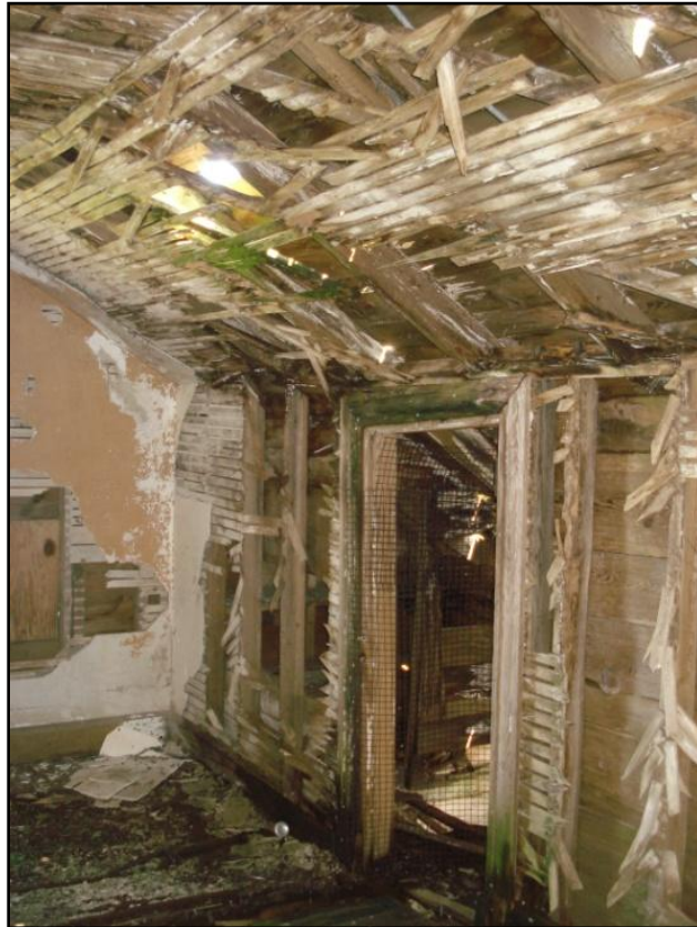
Figure 6: Interior damage to wooden elements
