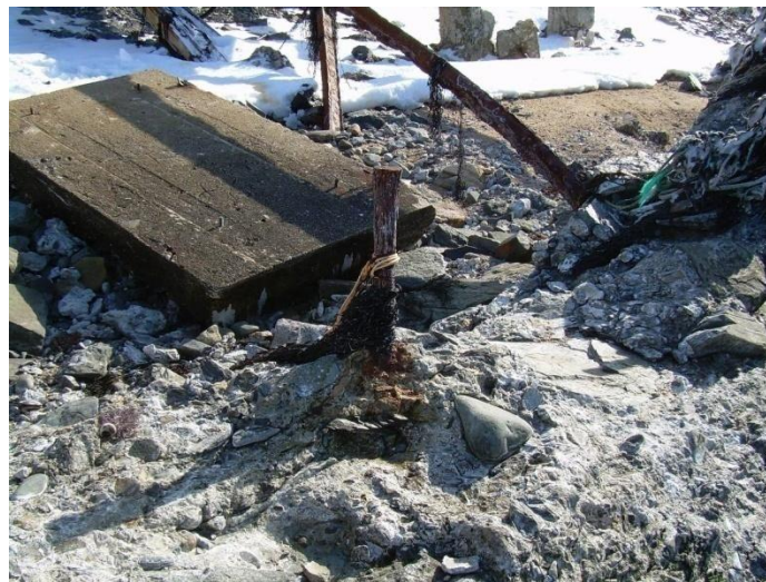
Figure 44: Corrosion of Tie Anchors along North Seawall (1)
