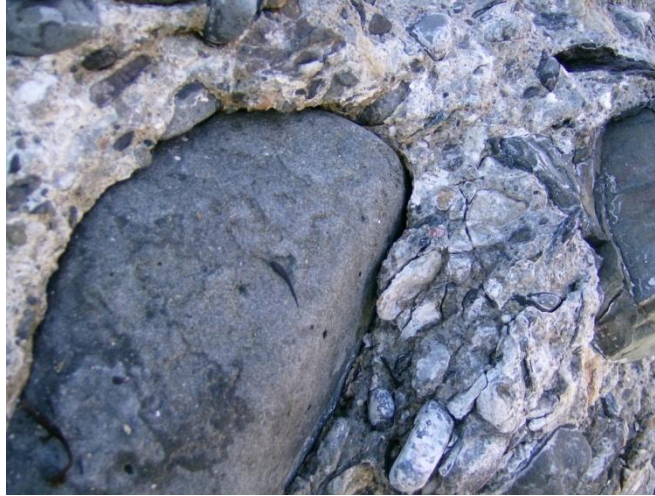
Figure 41: Un-bonding of Aggregate due to Freeze Thaw in North Seawall
