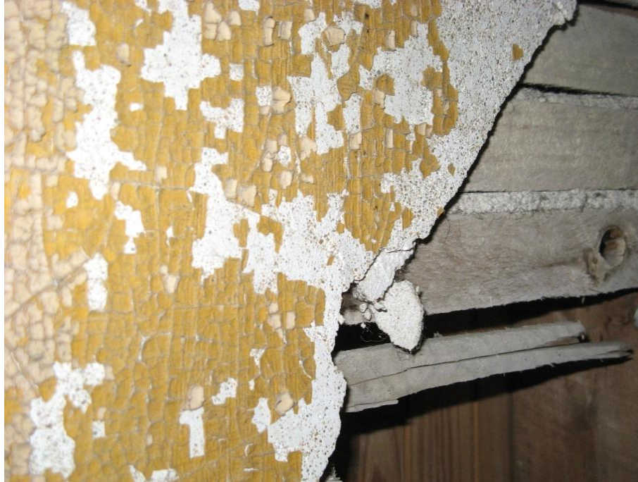
Figure 5: Lead paint chipping off interior walls
