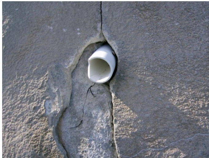
Figure 26: Weephole located halfway up on South Wall
