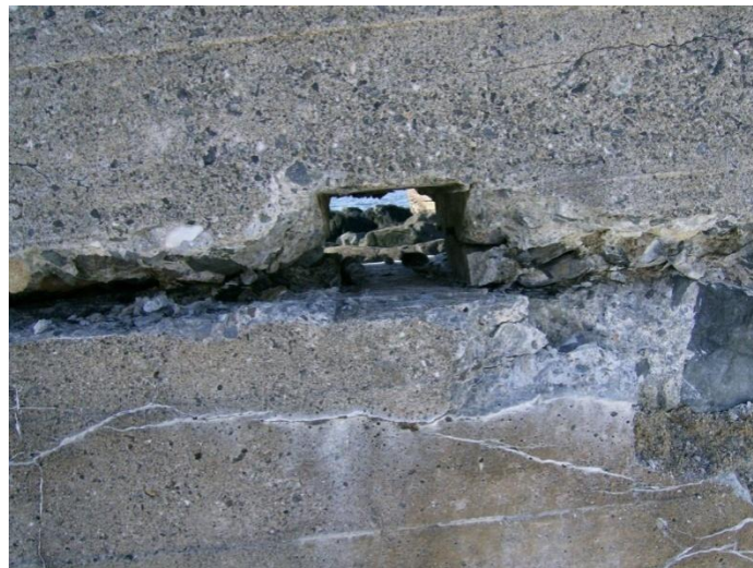
Figure 43: Cast in Place Drainage along North Seawall
