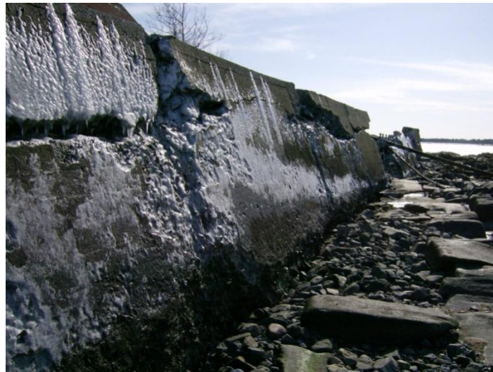
Figure 40: Visible Freeze Thaw on North Seawall
