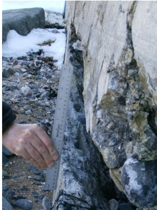
Figure 36: Horizontal Displacement and Overturning of North Seawall (1)
