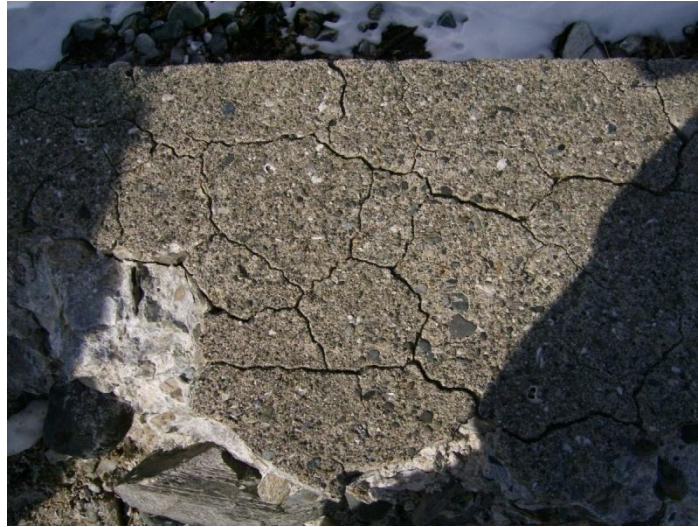
Figure 42: Spider Web Cracking Signs of ASR along North Seawall
