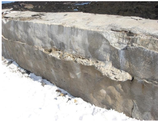
Figure 28: Signs of Backfill Weathering
