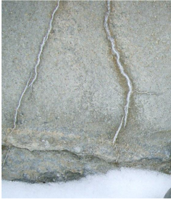
Figure 33: Leaching of Sulfates from South Seawall
