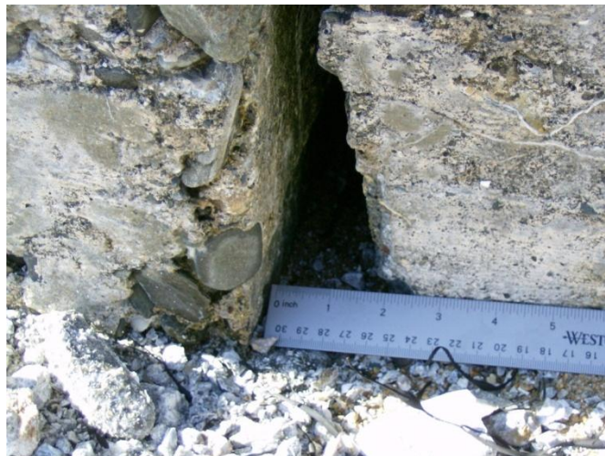
Figure 37: Horizontal Displacement and Overturning of North Seawall (2)
