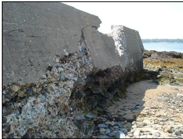
Figure 35: Undercutting of North Seawall (2)
