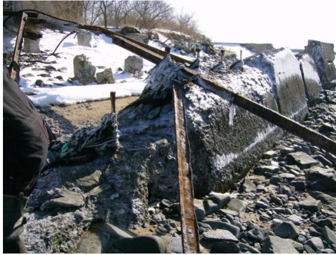
Figure 45: Corrosion of Tie Anchors along North Seawall (2)
