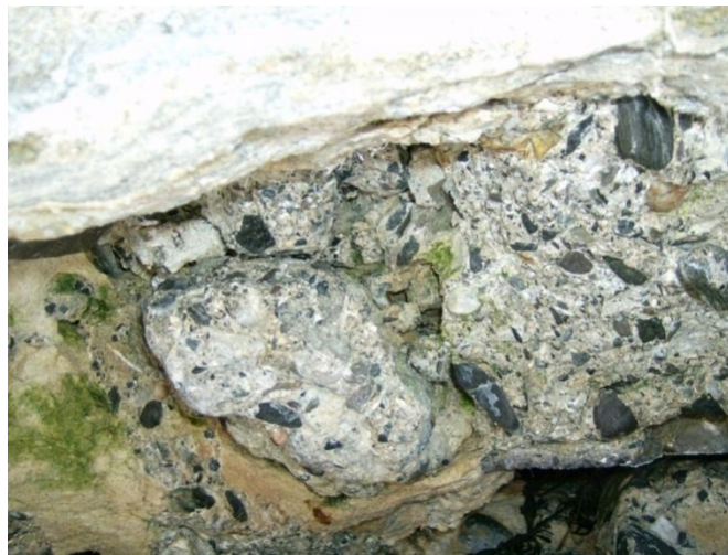
Figure 19: Undercutting of South Seawall
