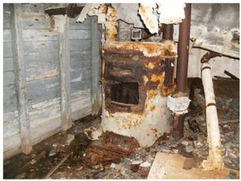
Presumed asbestos-containing boiler insulation and corrugated paper pipe insulation in the station basement.
