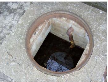
Looking into the concrete cistern showing the corroded metal pipe and accumulation of presumed rainwater.
