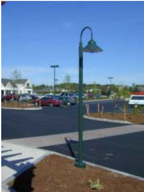
This pedestrian fixture has been located to illuminate the crosswalk that leads into a commercial establishment.
