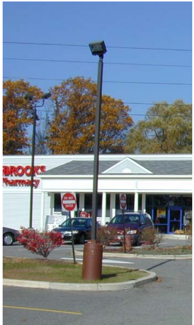
Spotlight fixtures should be avoided since they are difficult to aim and may cause spillover onto adjacent properties.
