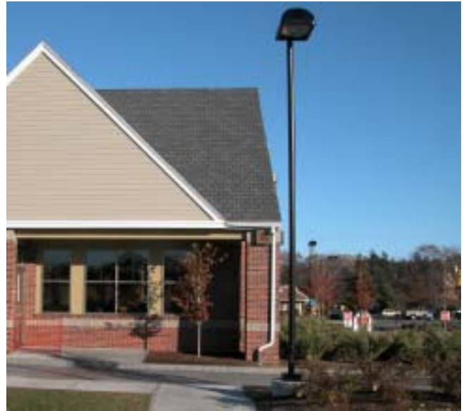
A cut-off fixture that complements the simple line of this commercial building. The fixture is mounted on an 18-foot pole on a one-foot base for an effective height of 19 feet.
